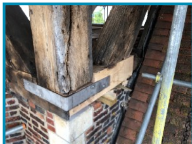
Photos of the Second Hard Hat Tour, New strengthening joints.
